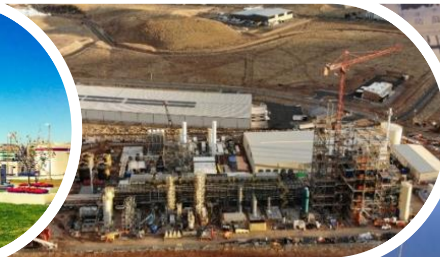
Sierra Biofuel Plant
