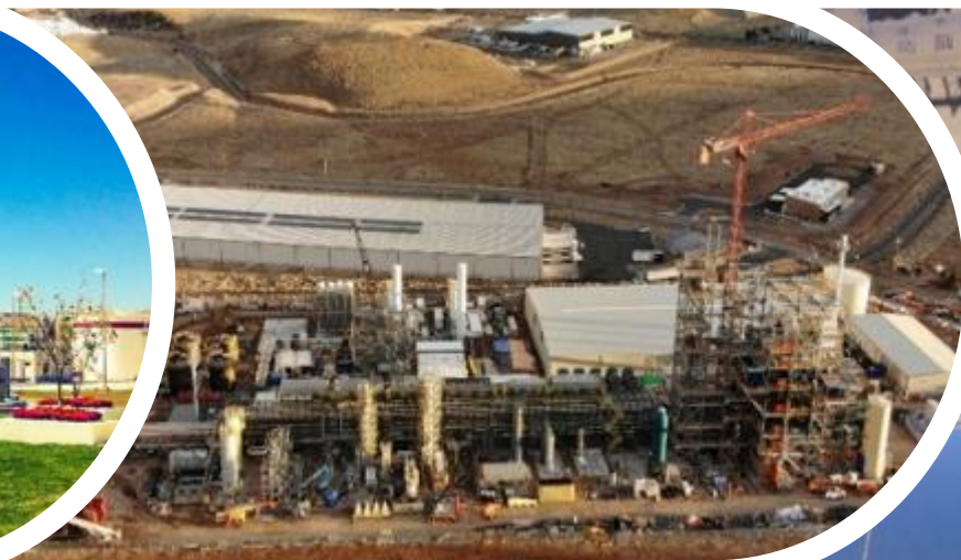
Sierra Biofuel Plant
