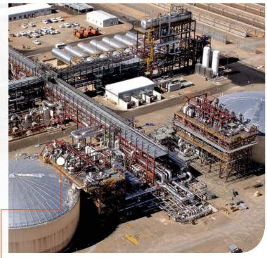
Components: Mirrors, collector assembly; perimeter fence/grading, pond; thermal storage foundation; steel tanks; substation/transmission lines; IT controls; feed water vessels; pump motors; heat transfer fluid and pumps; pressure heaters; thermal storage equipment; receiver tubes; ball joint assemblies; water treatment equipment; collector foundations; cooling/condensing system; night HTF pumps; hydraulic drives.
