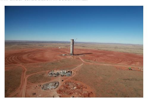
Khi Solar One, a 50 MW tower plant with 2 hours of steam storage, using superheated air and a dry cooling system to reduce water consumption; also, KaXu Solar One, a 100 MW parabolic trough plant with 3 hours of storage in molten salts.
