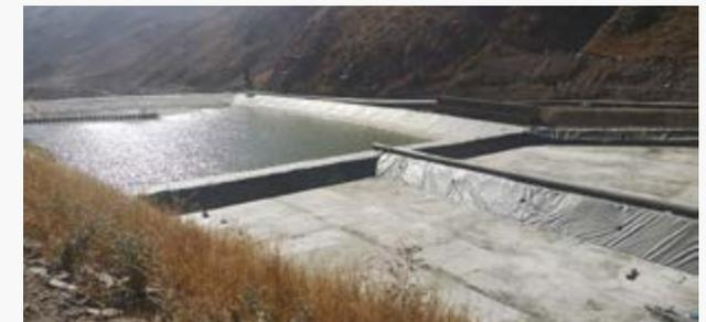
► 30,000 m<sup>3</sup> capacity retention dam reservoir built by Abengoa for the Cuajone mine.
