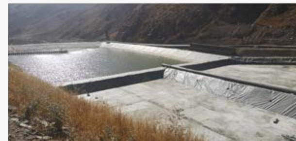
► 30,000 m<sup>3</sup> capacity retention dam reservoir built by Abengoa for the Cuajone mine.
