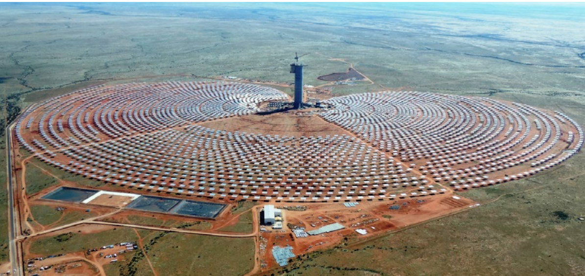
Khi Solar One, in South Africa, is one of the world's largest power tower plants
