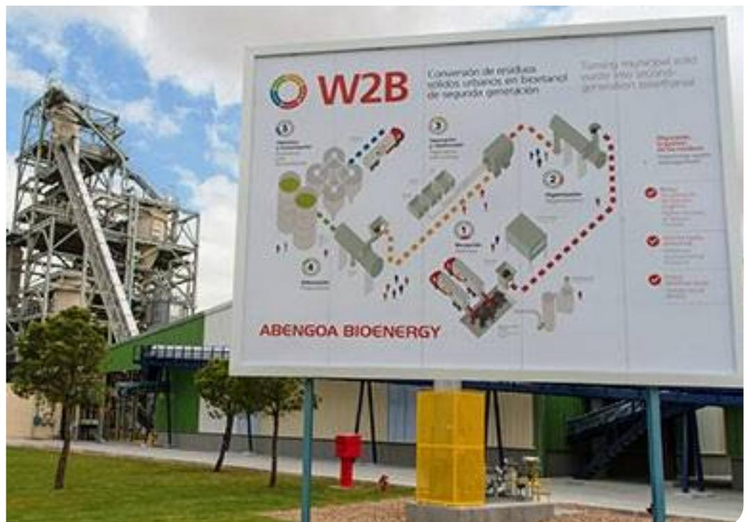
The W2B project is currently in the demonstration phase, for which purpose the biomass biorefinery located in Babilafuente (Salamanca) has been modified to be able to also process MSW and thus validate the complete ethanol from organic waste production chain. The operation of the demonstration plant provides valuable information for the design and subsequent operation of the commercial plant, thereby permitting the industrialization of this technology.
