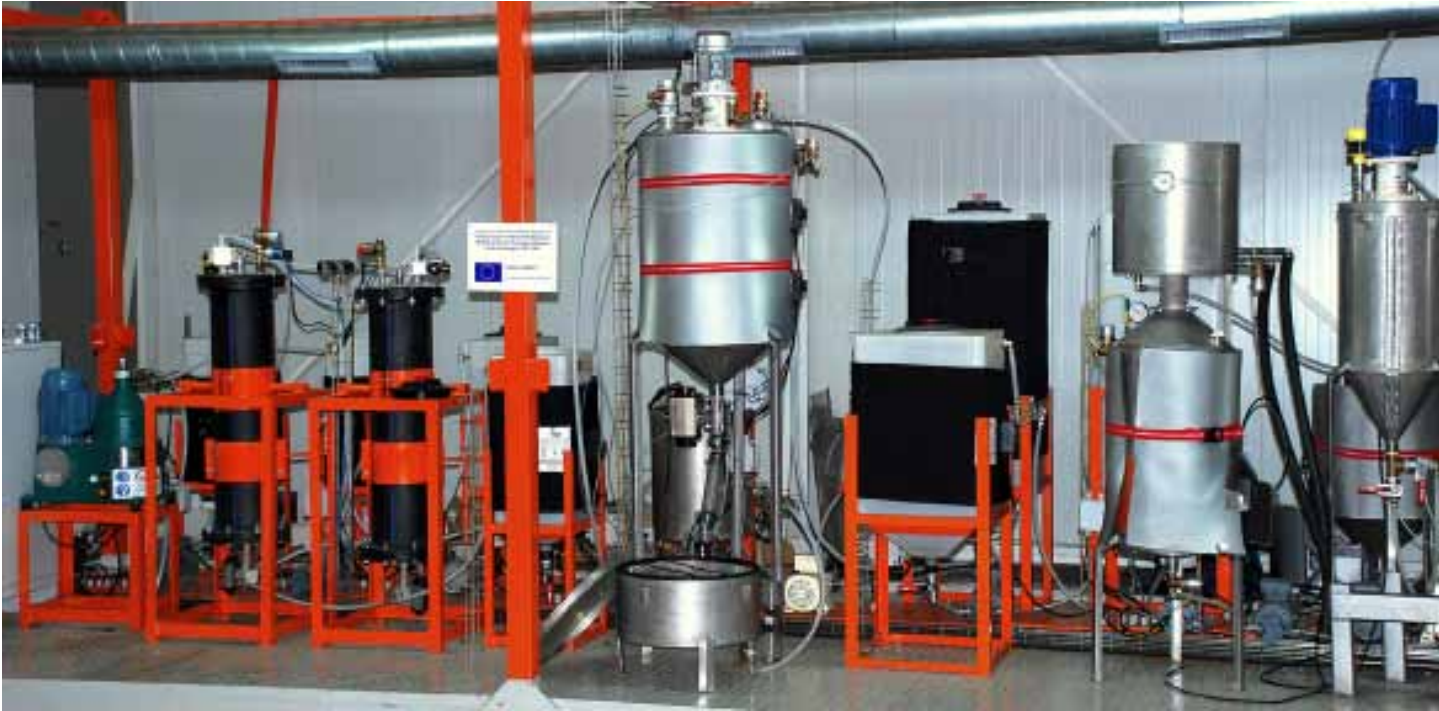
Glycerin etherification pilot plant
