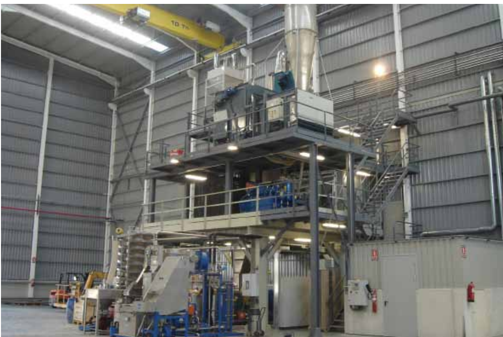
Fiberglass-reinforced plastic demonstration plant
