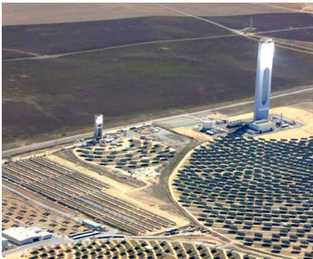
Aerial view of the Solucar platform (Seville, Spain), with some of the R&D&I facilities visible
