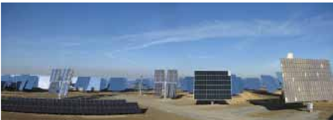
Different concentrating photovoltaic systems
