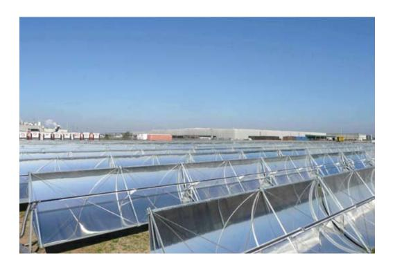
Industrial solar thermal installations employ parabolic trough technology, which not only produces electricity but is also ideal for generating thermal energy (heat and steam) for industrial processes. The main advantage that this technology offers is that it can be adapted to different needs, while also helping to cut  $\mathsf{CO}_2$  emissions, given that industry is one of the primary sources of these gases.
