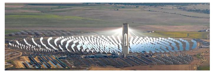
Its solar field, with 624 heliostats of 120 m<sup>2</sup> each, is particularly eye-catching. It concentrates solar radiation onto the receiver that is located at the top of a 120 m high tower to produce steam and drive a turbine coupled to the electrical generator connected to the power grid.
