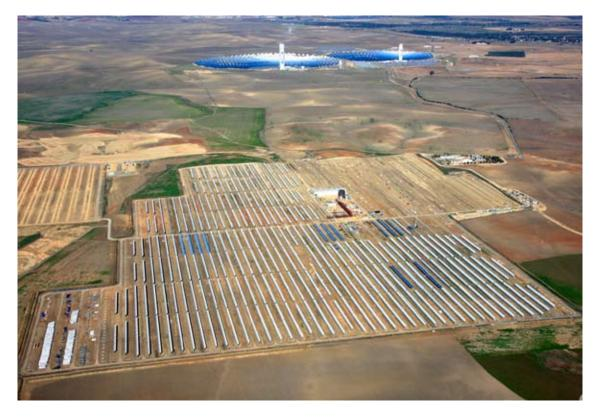
The technology consists of concentrating solar radiation by means of high-precision curved mirrors onto a heatabsorbing pipe, inside which circulates a fluid that reaches high temperatures. This fluid enables the production of steam that is sent on to a turbo-generator, where it expands in order to produce energy.
