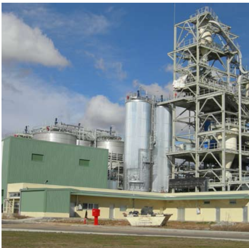
Enzymatic hydrolysis biofuel demo plant in Castilla y León.
