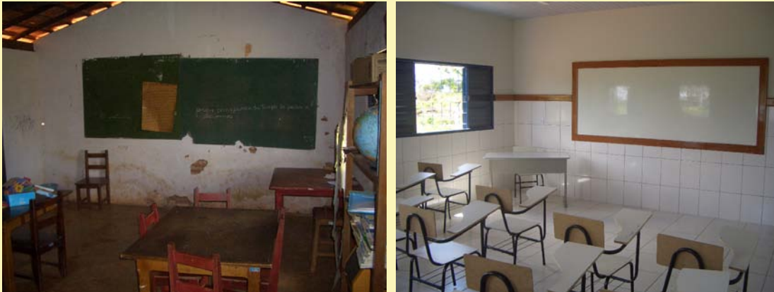
Before and after rebuilding the Santa Clara Municipal School
