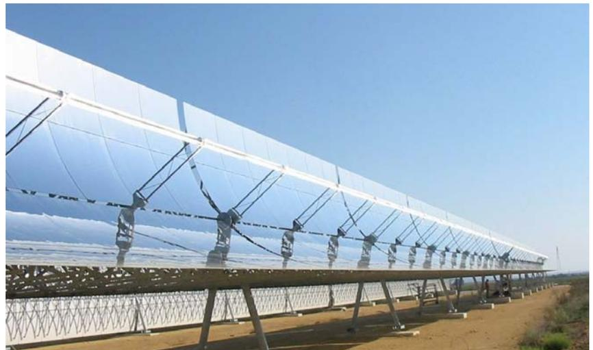
**First Integrated Solar Combined Cycle (ISCC) plant, in Algeria**
