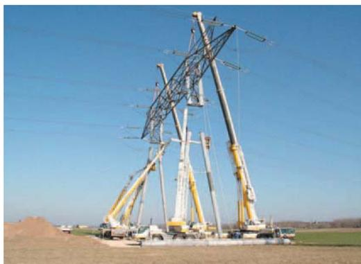
As regards execution, works of very different natures were executed during the year, of note among which is the heightening of a stay portico on the 400 kV Dambron-Verger line, which was done in the presence of a large number of technical experts from RTE to their complete satisfaction, and the company was congratulated on the works by the customer.
