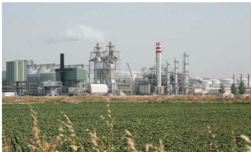
pressure steam, followed by enzymatic hydrolysis with celluloses and subsequent fermentation of the sugars liberated with commercially available yeasts. Plant production capacity is 5 million liters per year of bioethanol.
