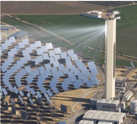
**Operating principle:** A circular array of heliostats (2 axis tracking mirror) is used to concentrate sunlight to a central receiver mounted on the top of a tower. A heat transfer medium in this receiver absorbs the highly concentrated radiation and converts it into thermal energy to be used by a turbine.
