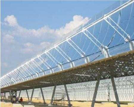
**Operating principle:** Parabolic troughs are used to track the sun and concentrate sunlight on to the thermally efficient receiver tubes placed in the trough focal line. In these tubes, a thermal transfer fluid is circulated, such as synthetic thermal oil. This oil is then pumped through a series of heat exchangers to produce steam. The steam is converted to electrical energy in a conventional steam turbine generator.
