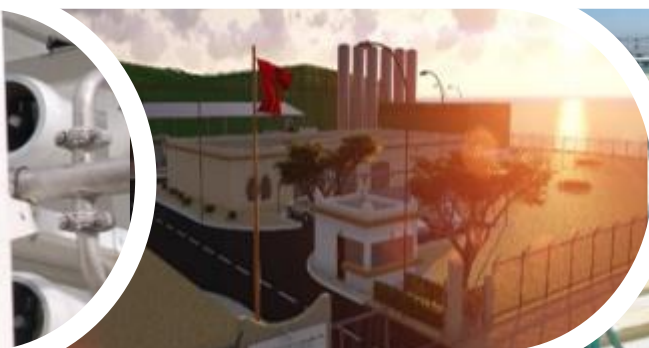
Agadir desalination plant Morocco
