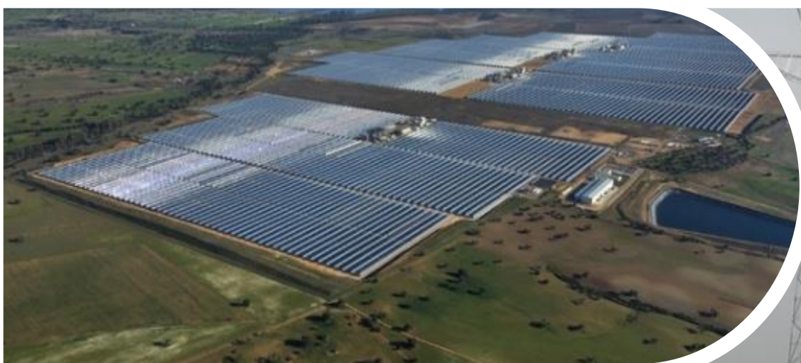
Solar thermal plants
