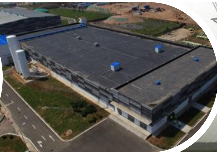
Qingdao desalination plant
