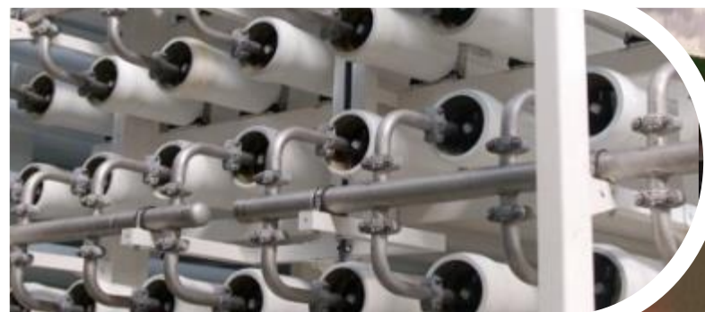
Taweelah desalination plant United Arab Emirates
