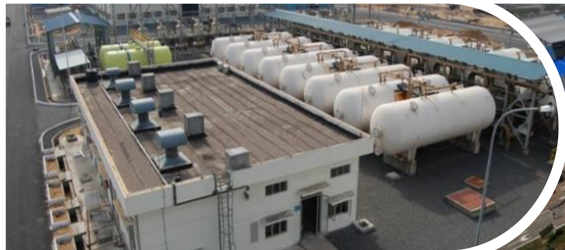
Chennai desalination plant
