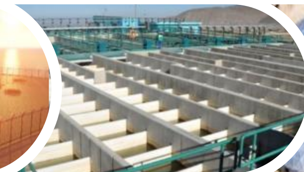
Cunene supply and sanitation system Angola
