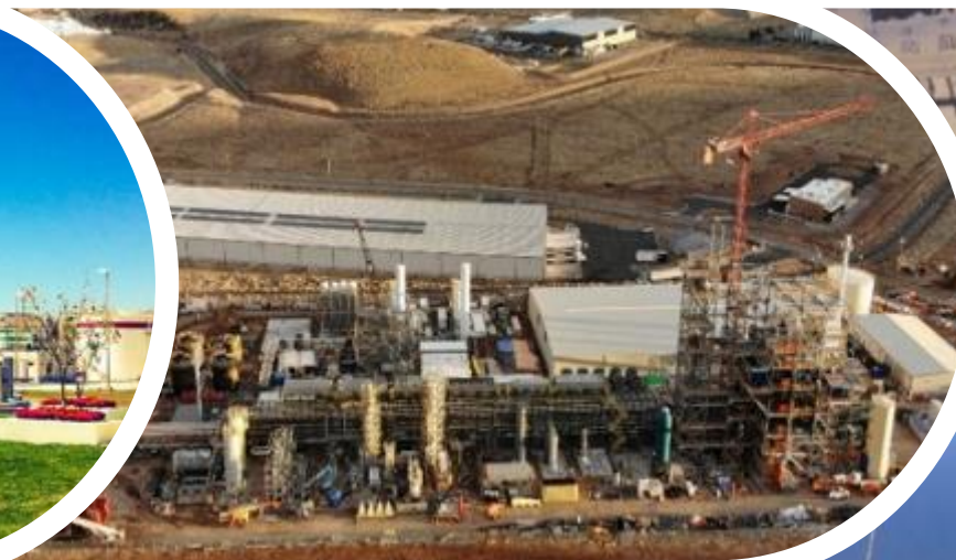
Sierra Biofuel plant
