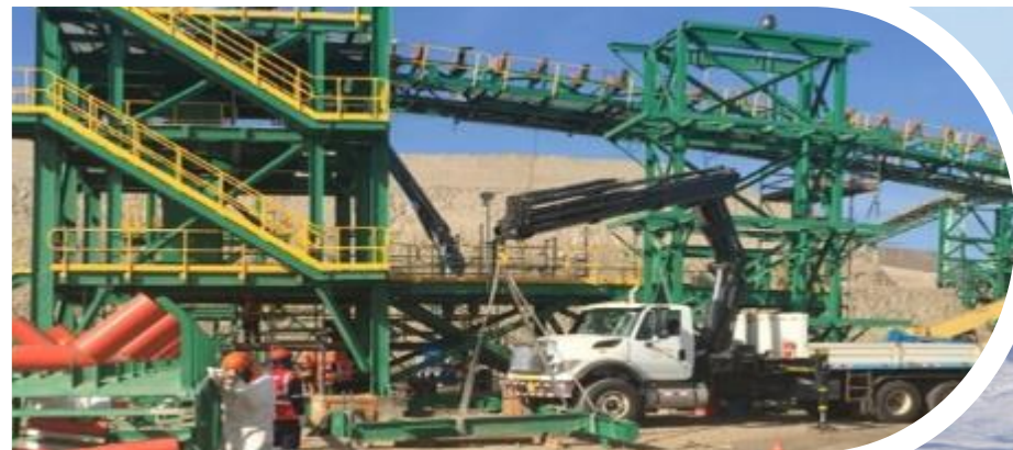
Shougang Mine extension packages 4 and 5
