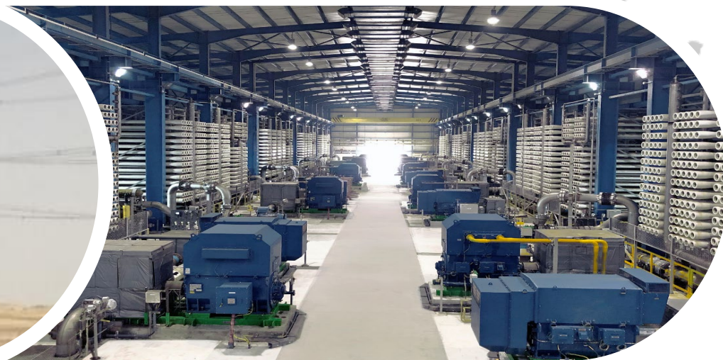
Shuaibah Desalination Plant
