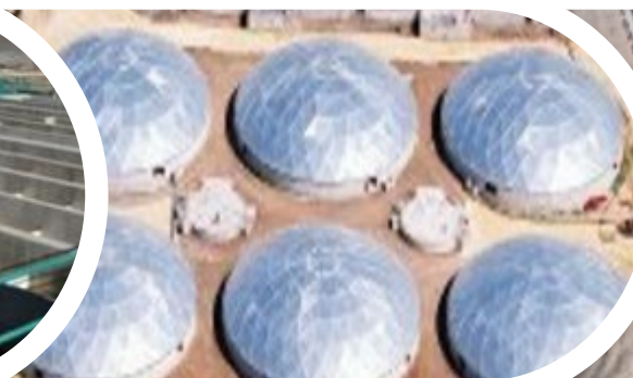
Sewage treatment plant Ranilla Spain
