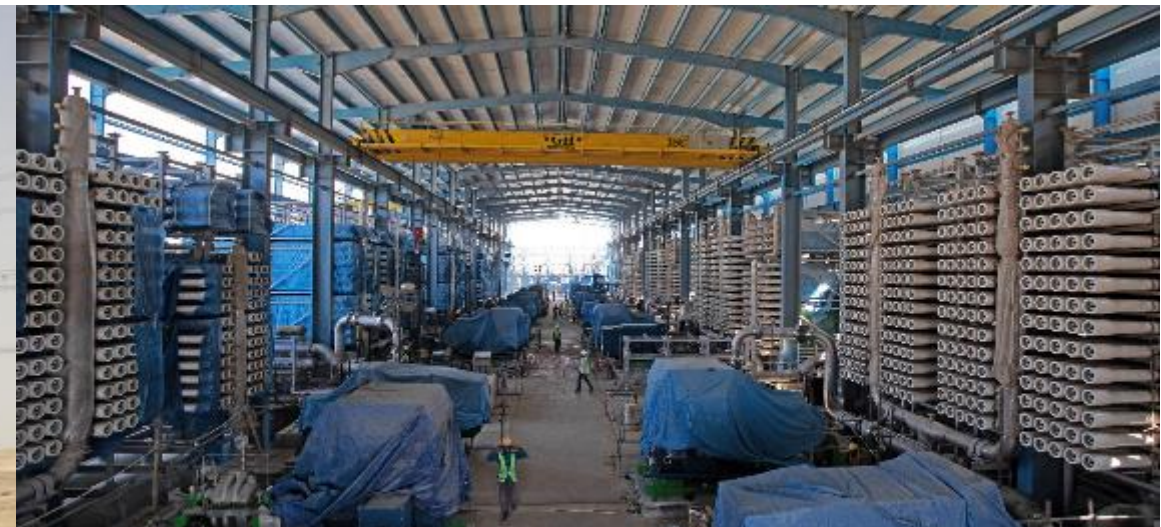
Shuaibah Desalination Plant Saudi Arabia
