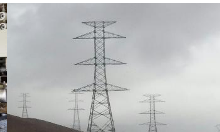
225 kV Line Morocco
