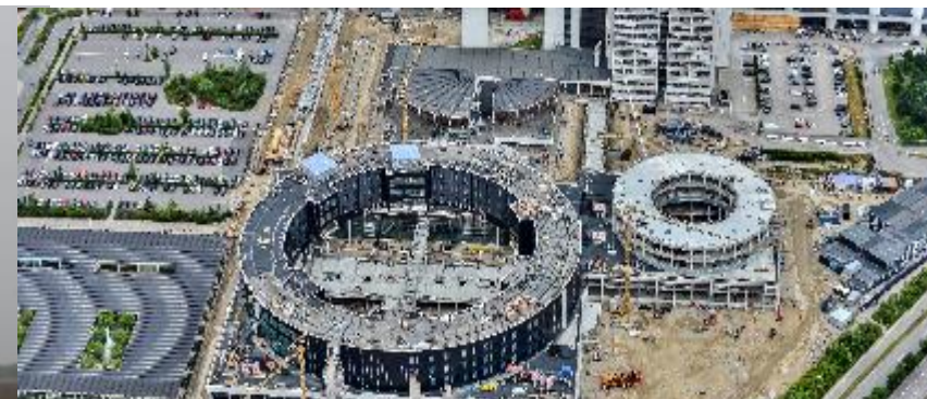
Electromechanical installations Denmark
