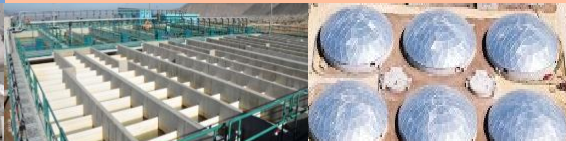
Cunene supply and sanitation system Angola
