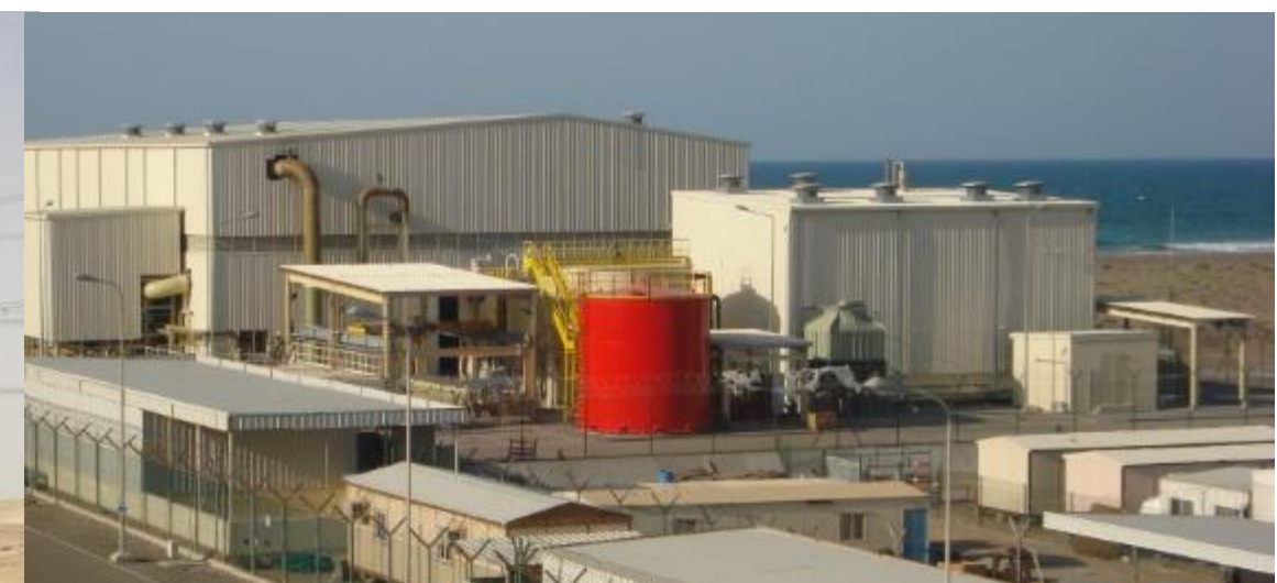
Barka Desalination Plant Oman
