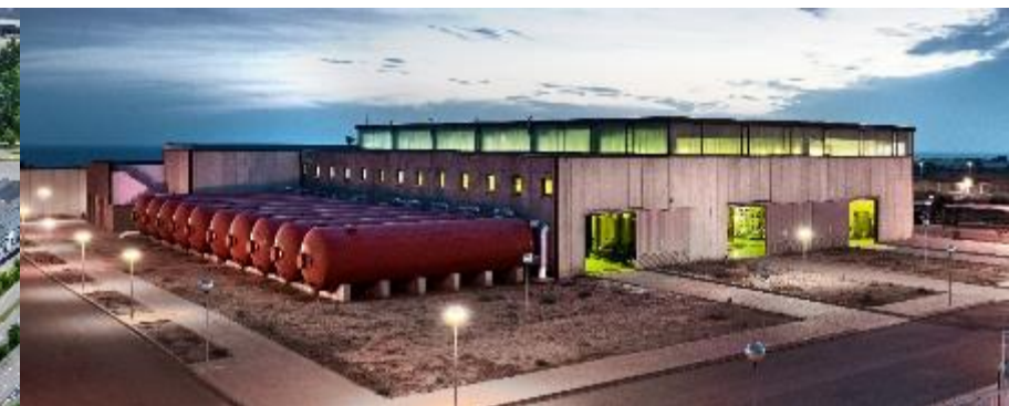
Desalination plants Spain
