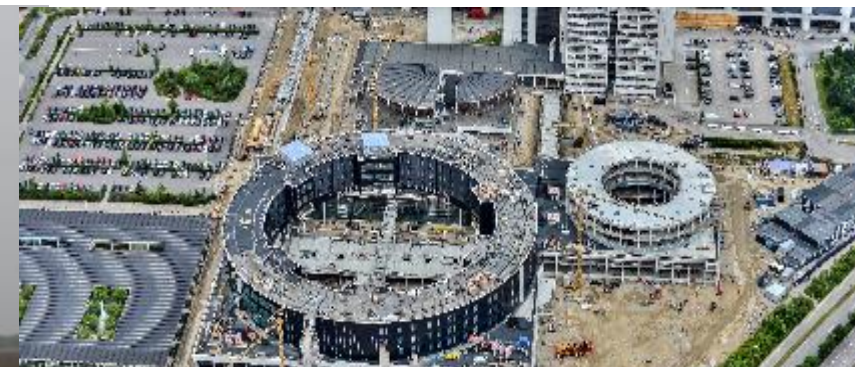
Electromechanical installations Denmark
