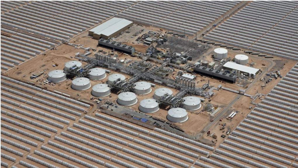
Abengoa successfully operated a thermal storage demonstration plant using molten salts, which was then commercialized at Solana. The storage system provides six hours of thermal storage at maximum capacity.
