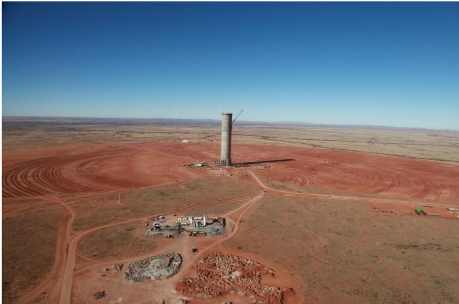
Khi Solar One, a 50 MW tower plant with 2 hours of steam storage, using superheated air and a dry cooling system to reduce water consumption; also, KaXu Solar One, a 100 MW parabolic trough plant with 3 hours of storage in molten salts.
