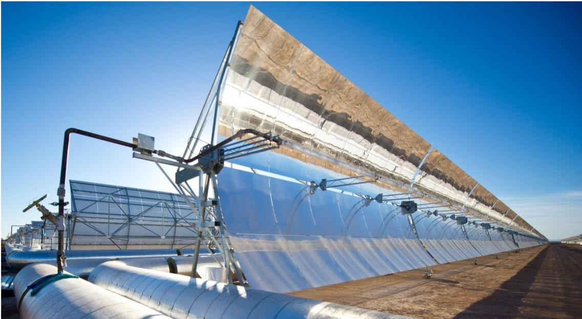
The parabolic trough technology is a mature and viable solution, with more than 25 years of proven operation experience with the launch of the first parabolic trough plants in the US (Solar Energy Generating Systems in California).
