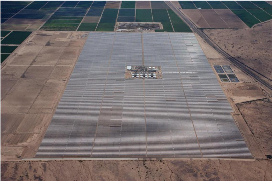
Solana, the largest parabolic trough technology plant in the world, has a gross capacity of 280 MW and six hours of storage, enabling it to satisfy the peak demand in this region in the late summer evenings and night time hours. Its solar field covers 3 mi<sup>2</sup> with approximately 3,200 mirrored parabolic trough collectors.
