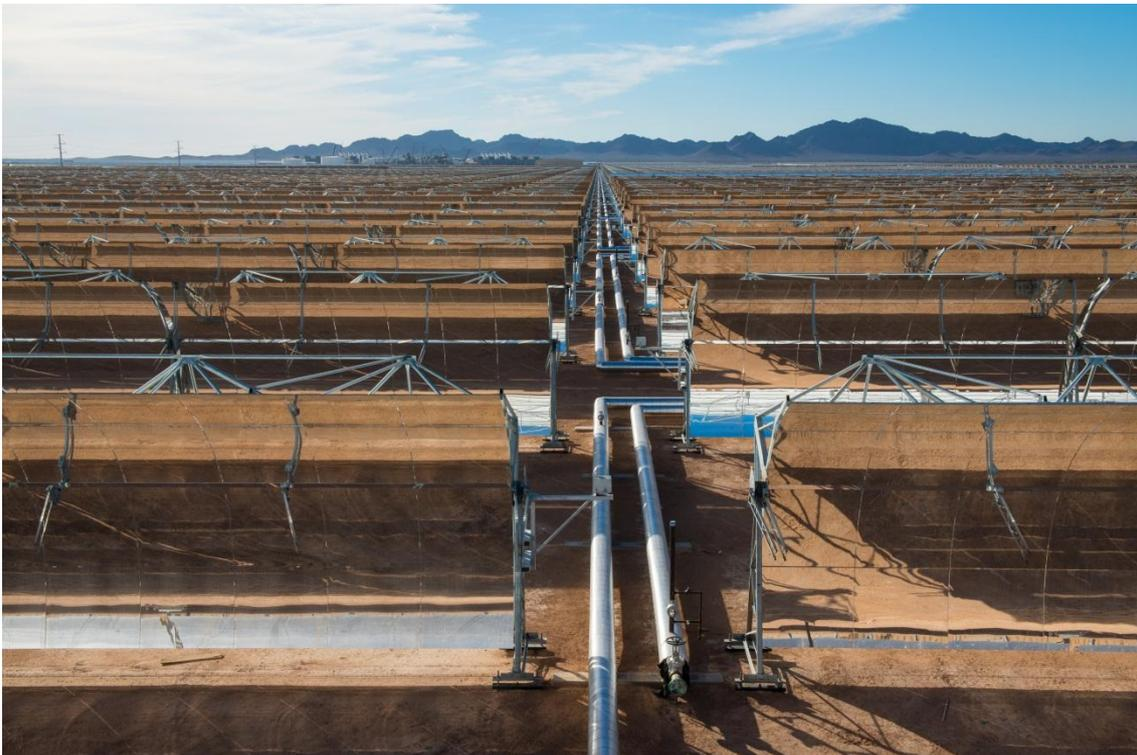
➤ **Parabolic trough collector technology**
