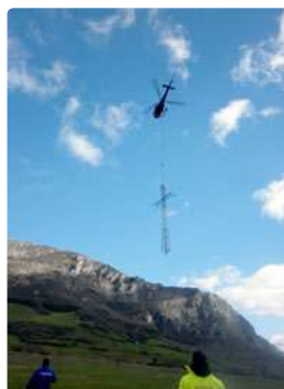
Installation of the tower for the deployment of the fibre-optic network in Navarra.
