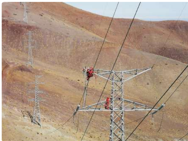
Repowering the Maitencillo Caserones transmission line.
