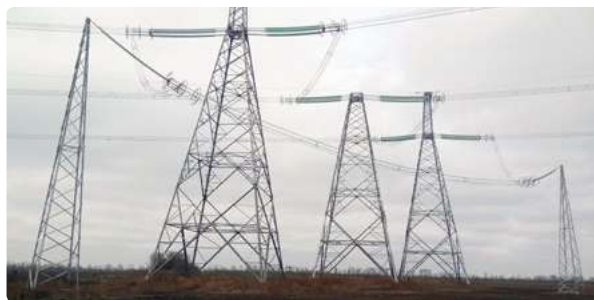
Construction of a 765-kV line with a length of 187 km in Ukraine.
