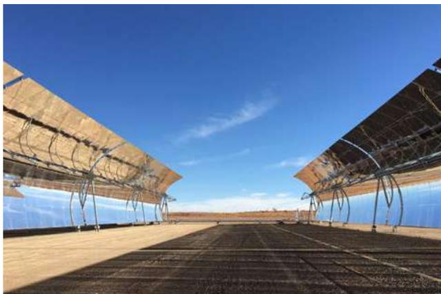
Large-aperture collector installed in Xina.
