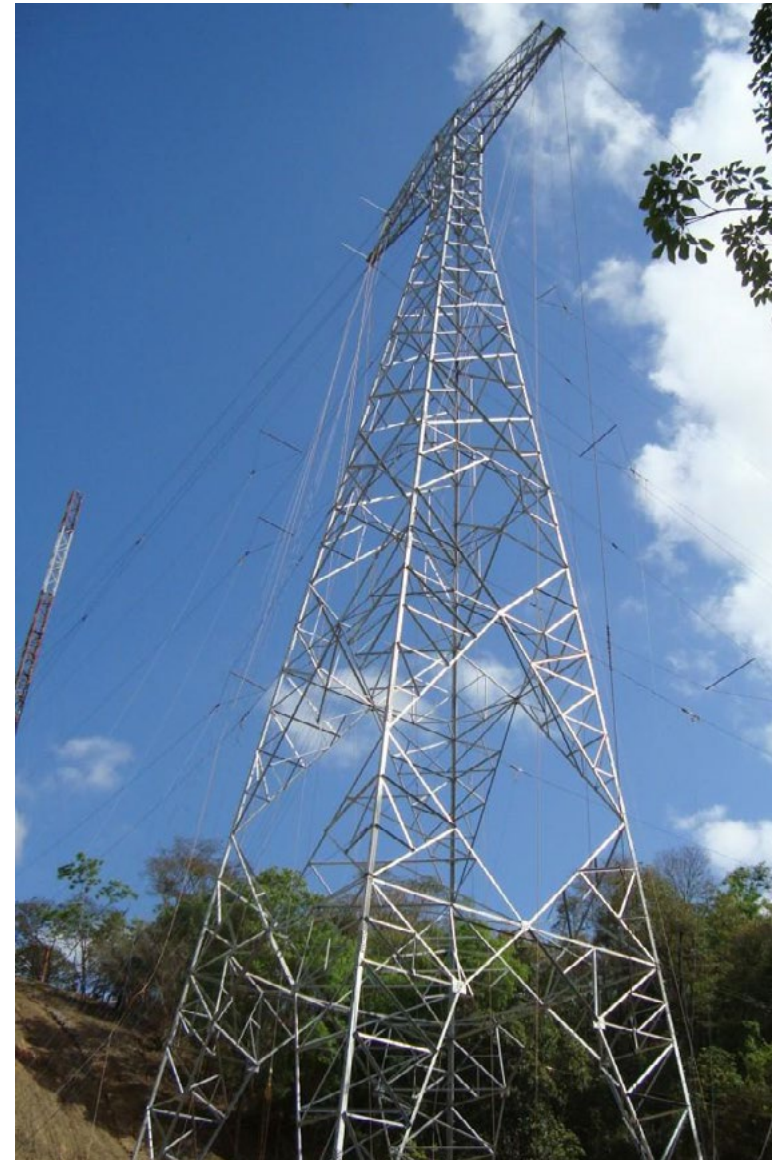
Abengoa has brought the world's longest direct current power line online
