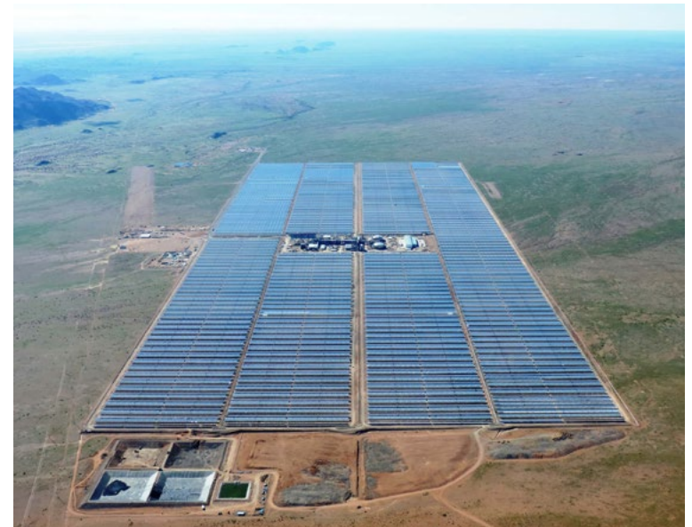
Construction of KaXu Solar One was completed in 2014 and the plant will begin operating commercially in early 2015
