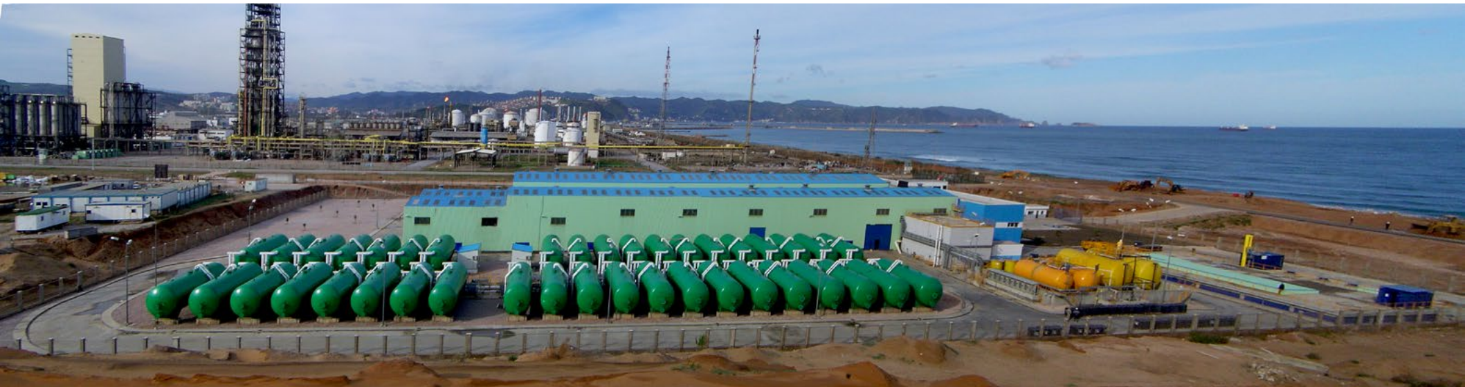
The Skikda desalination plant (Algeria), with a capacity of 100,000 m 3 /day, has been in operation since 2009
