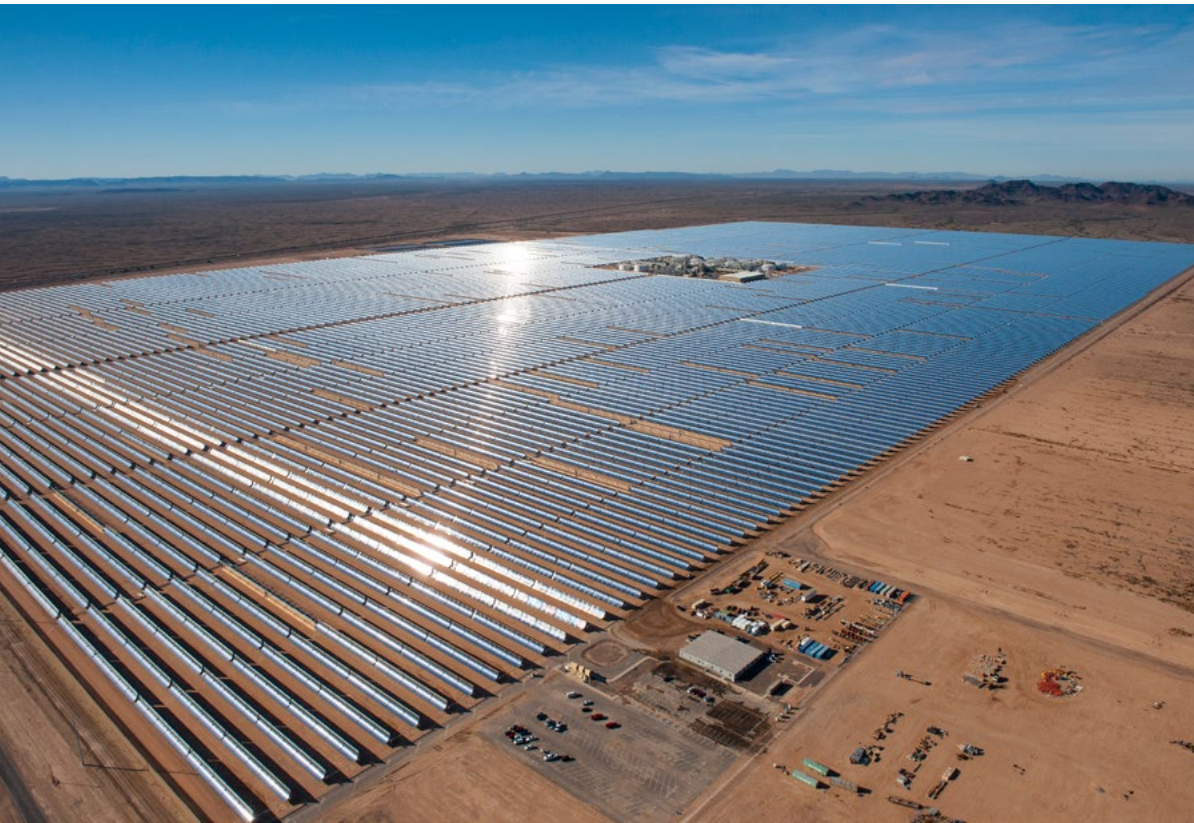
Solana, with an installed capacity of 280 MW, is the world's largest parabolic trough facility.
