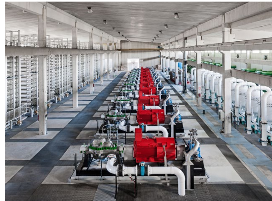
The Cartagena desalination plant (Spain), with a capacity of 65,000 m 3 /day, has been in operation since 2005
