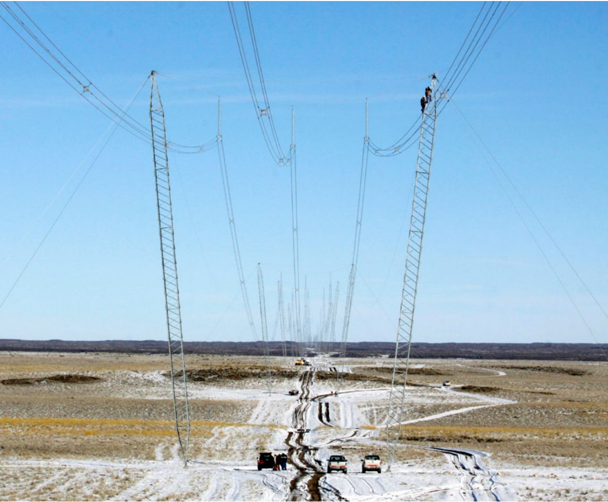
Transmission line in Argentina, where Abengoa built its first transmission line outside Spain
