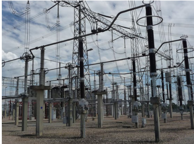
Abengoa has built 284 substations in the last 10 years
