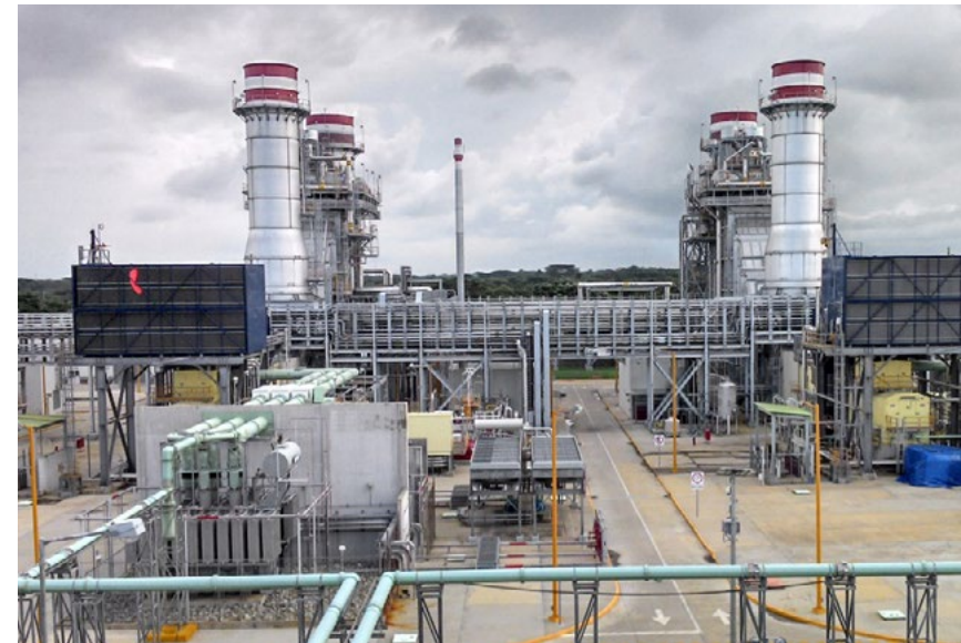
Abengoa has more than 9 GW of installed capacity in conventional generation
