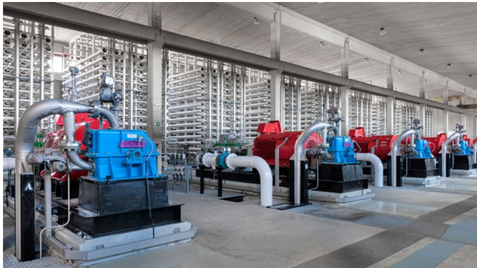
Desalination plant at Cartagena, Spain, with an installed capacity of 65,000 m 3 /day and featuring reverse osmosis technology
