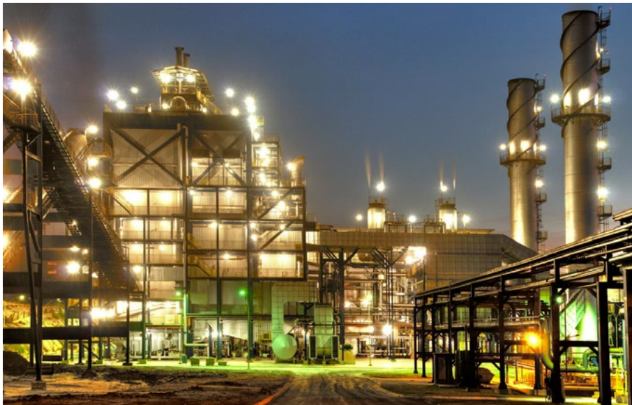
Electricity cogeneration at Abengoa's plant in Sao Luiz (Pirassununga, Sao Paulo, Brazil)
