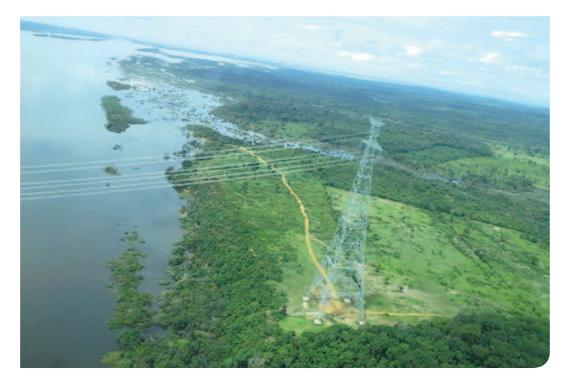
Itacayunas-Carajás (ATE VIII), 130 km and 230 kV. Located in the state of Pará in northern Brazil, it supplies the 150,000 inhabitants of Parauapebas. The transmission line provides greater reliability to local industries, in a region with some of the highest levels of mining activity in Brazil. Abengoa has a 30-year concession.
