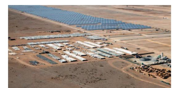
Hassi R'Mel, the 150-MW integrated solar combined cycle (ISCC) plant with parabolic trough solar field is located in Algeria.
