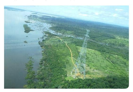
Itacayunas-Carajás (ATE VIII), 130 km and 230 kV. Located in the state of Pará in northern Brazil, it supplies the 150,000 inhabitants of Parauapebas. The transmission line provides greater reliability to local industries, in a region with some of the highest levels of mining activity in Brazil. Abengoa has a 30-year concession.
