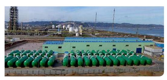
Honaine: The purpose of this desalination plant is to produce drinking water from seawater to supply the city of Honaine, Tlemcen. The plant supplies a population of almost one million. It has a capacity of 200,000 m<sup>3</sup>/day and has been operating since 2011.
