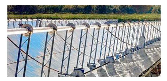
The facility consists of two independently constructed and operated parabolic trough plants. Both plants are jointly owned by Abengoa and the Japanese conglomerate JGC. Abengoa operates both plants and has a 74 % stake.
