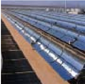
Parabolic trough
