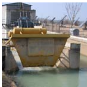
Mini hydro station sluice gate to keep water levels constant on the Aragon and Catalonia Canal.
