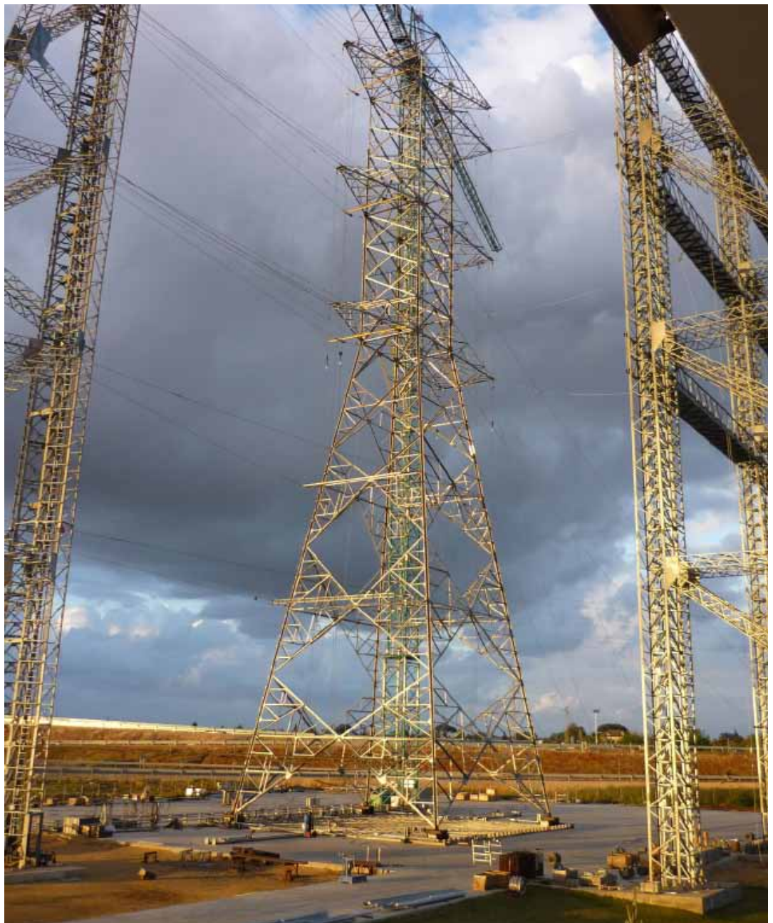
Tower designed and constructed by Comemsa
