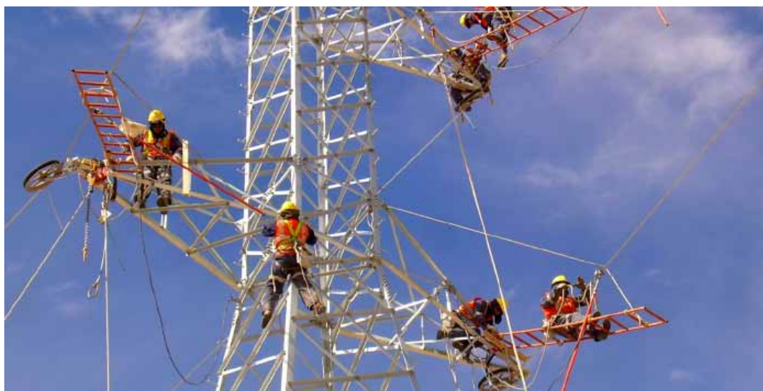
Workers constructing a power transmission tower in Chile
