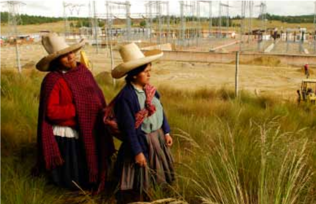
Peasants next to the Cajamarca substation on the 220 kV Carhuamayo-Carhuaquero transmission line in Peru
