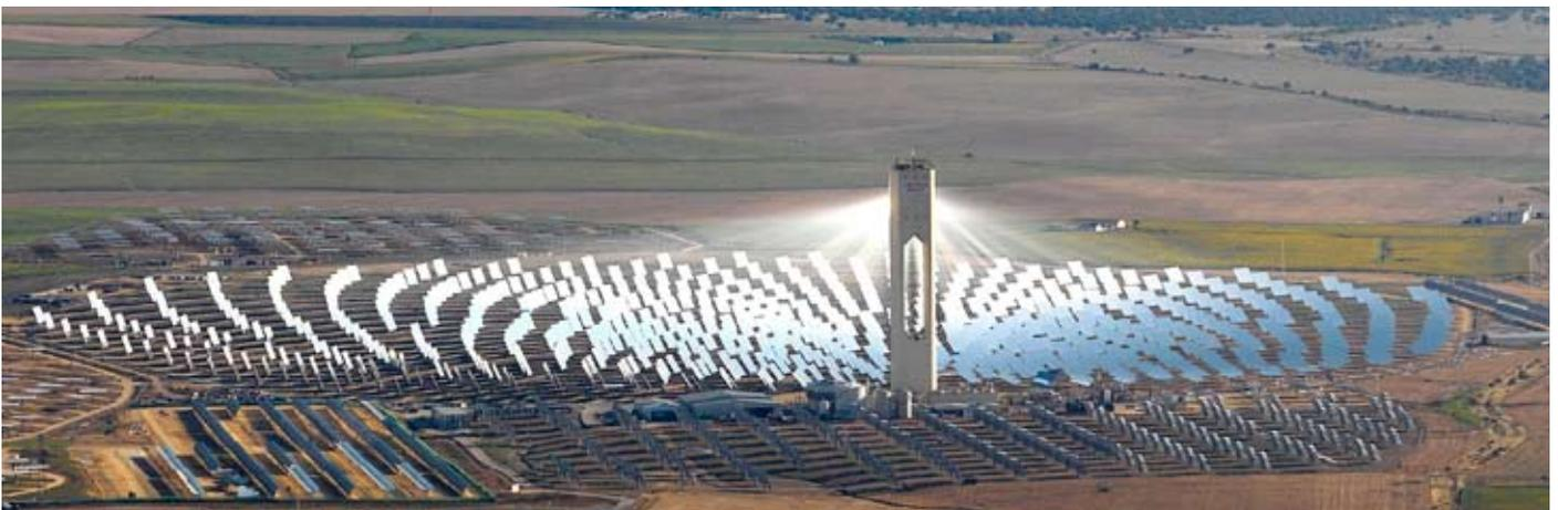
Its solar field, with 624 heliostats of 120 m<sup>2</sup> each, is particularly eye-catching. It concentrates solar radiation onto the receiver that is located at the top of a 120 m high tower to produce steam and drive a turbine coupled to the electrical generator connected to the power grid.
