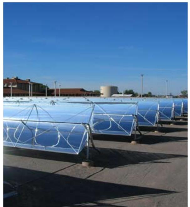
The collectors will operate at temperatures of up to 250 °C to produce steam. This steam is then transferred to a plant where it is used to heat the oil for frying potato chips and other snacks.
