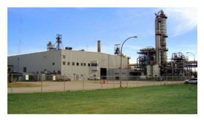
The  ${\rm CO_2}$  produced is captured and refined by an on-site customer. The produced DGS is not dried in the process; 100% of the co-product is sold in its natural state. Corn and sorghum can be employed simultaneously, although the primary raw material is sorghum, and more than 50% of the plant's energy requirements are provided by methane from a municipal solid waste landfill. It currently employs 48 highly qualified professionals.
