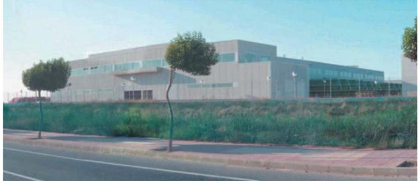
Bajo Almanzora (Almeria) desalination plant. The contract includes its construction, operation and maintenance for 15 years. The plant's desalination process will be reverse osmosis and it will be provided with the most efficient energy recovery technology currently available: isobar chambers. A total of 15 municipalities and more than 12,031 hectares of agricultural land will benefit from the plant's 60,000 cubic meter per day production capacity.
