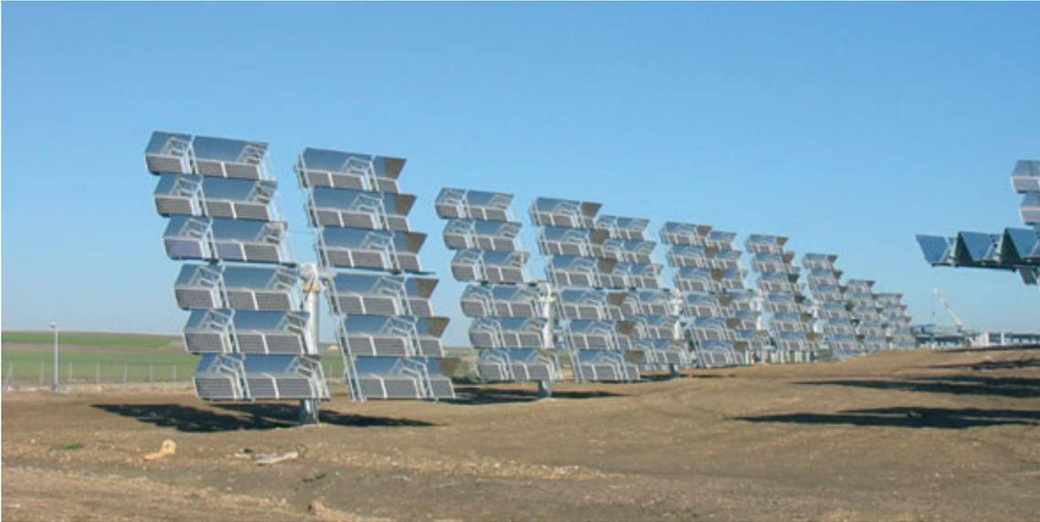
This project represents the launching, following several years of research and development by Abengoa, of the electricity harnessing technology for the renewable solar resource known as tower and heliostat field technology. The main contribution of the PS10 project to the development of this technology lies in it being the first tower solar thermal power plant in the world that will produce electricity in a stable and commercial manner.
