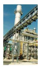
The principal characteristics are: production of 216,000 MWh/year of electrical power and consumption of 160,000 tons/year (20,000 Kg/hour) of biomass
